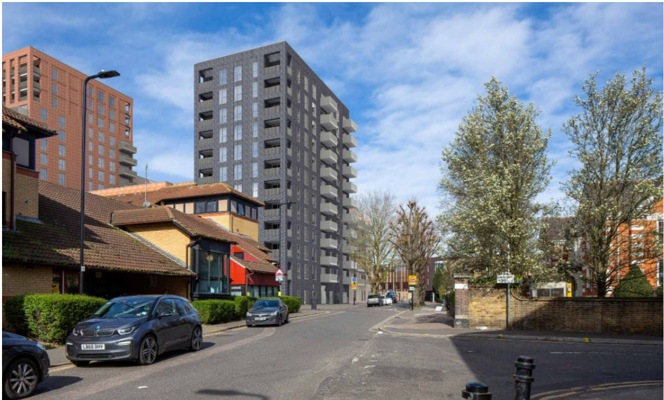
Figure 10: View of development from Green Man Lane
